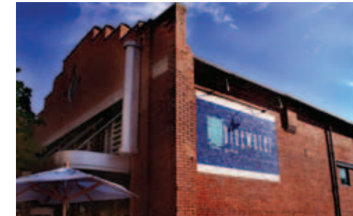
◀ Bluewater Grille restaurant, downtown Chattanooga. Interior remodel of existing trolley barns, circa 1906.
