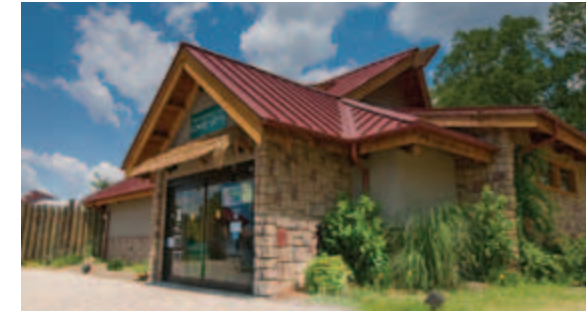
▲ Gift Shop, Chattanooga Zoo at Warner Park. One of five new buildings of zoo expansion including pedestrian plaza, carousel/concessions building and administration building. 2006.
